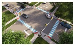
include reducing vehicular travel lanes from two in each direction to one in each direction with a center turn lane, new sidewalks, traffic signal upgrades, lighting improvements, landscaping improvements, and public art. Construction is expected to conclude by winter 2025.
